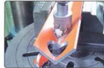
Angled steel boring
